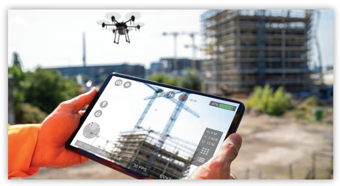
What's more, drones are expected to take on an even larger role in construction thanks to recent improvements. Today's models offer real-time aerial imagery and 3D lidar (Light Detection and Ranging) scans. They can also integrate with building information modeling software.
